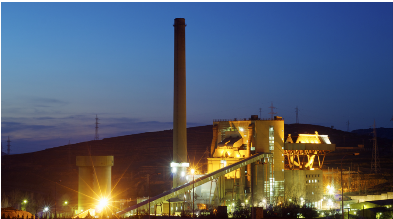
Factory production of electricity using coal, Teruel, Aragon, Spain
